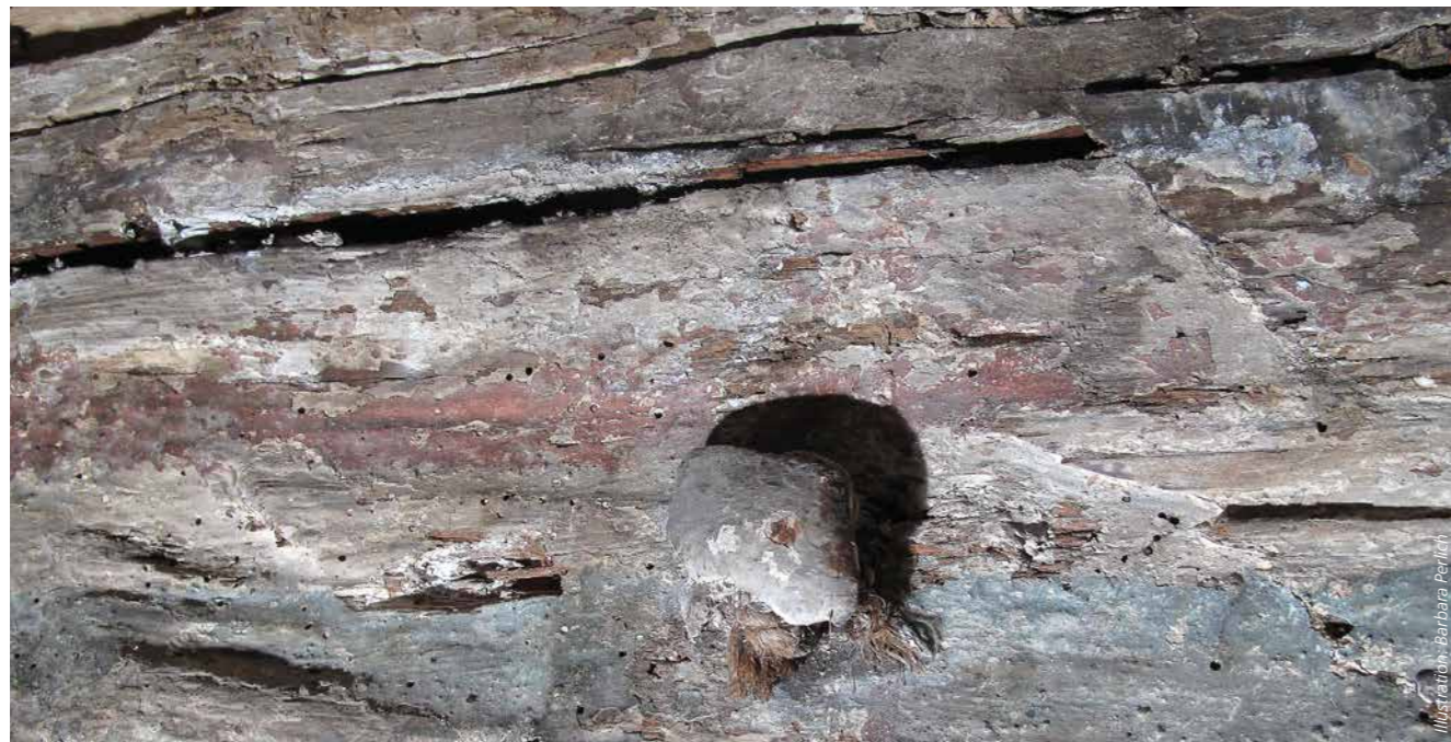
Lamps could be hung from the studs in the beams opposite the Torah cupboard (see illustration page 30/31).
