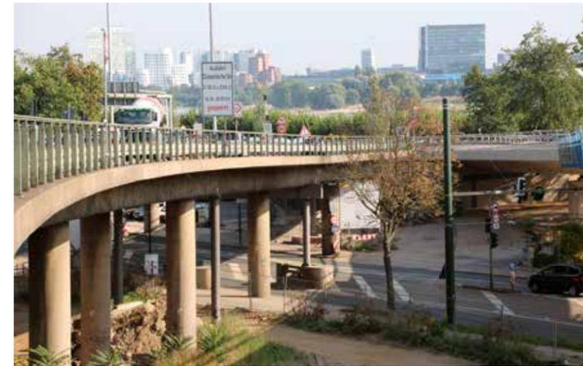
Left: Flyover of prestressed concrete in the Heerdter Dreieck in Düsseldorf shortly before it was dismantled. Below: A glimpse inside – exposed tendons with strain gauges; a tendon was cut through to simulate failure.
