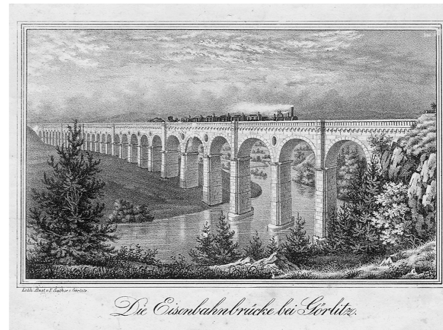
The Lusatian Neisse Viaduct, completed in 1847, was one of Silesia's largest rail bridges.
