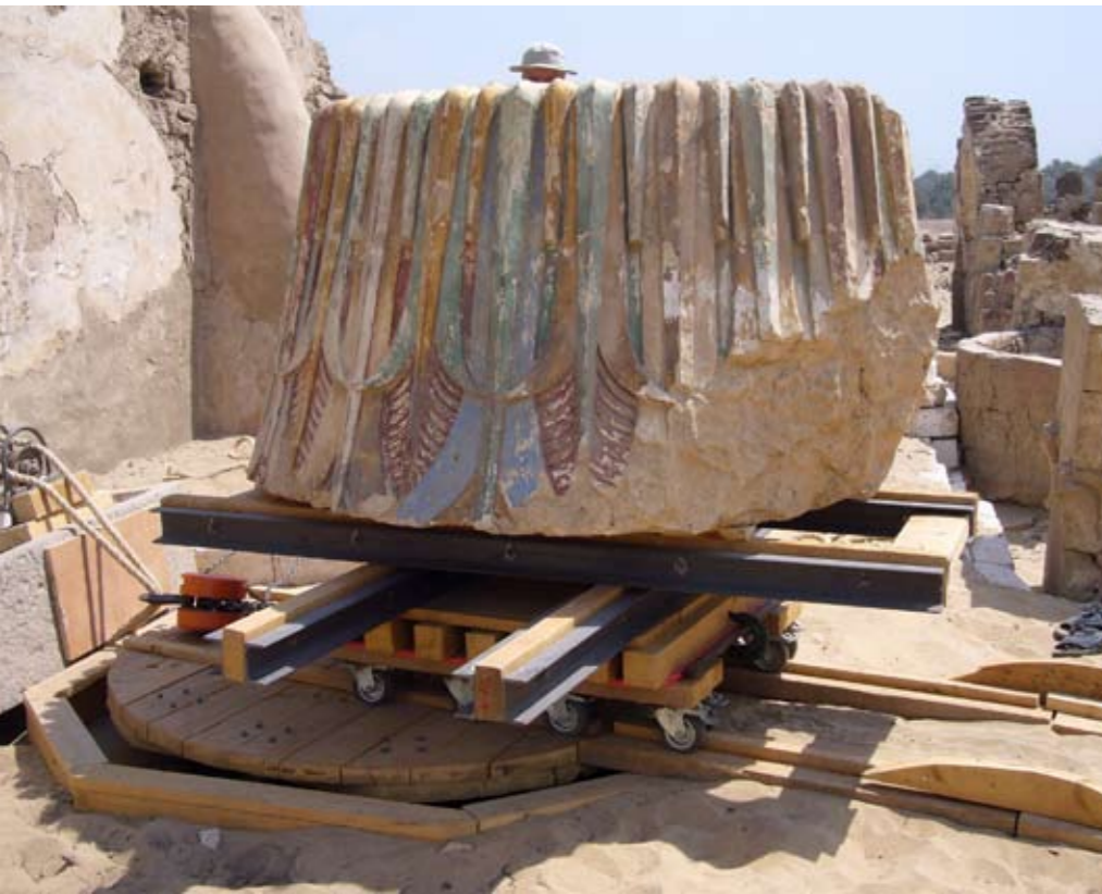
A multi-coloured capital fragment rests on a specially constructed turntable. This facilitates changes of direction during transportation.
