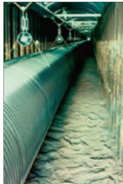
ed stainless steel tubes of 60 centimetres in diameter. The vacuum required here is similar to near-earth space.
