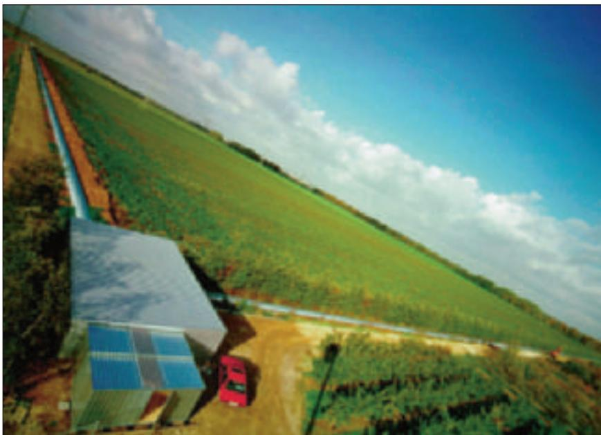
A bird's eye view of GEO600: Running from the main building are two 600-metre arms, each with its own terminal building. The arms themselves (right) are enclosed in stainless steel tubes that are suspended in trenches.
