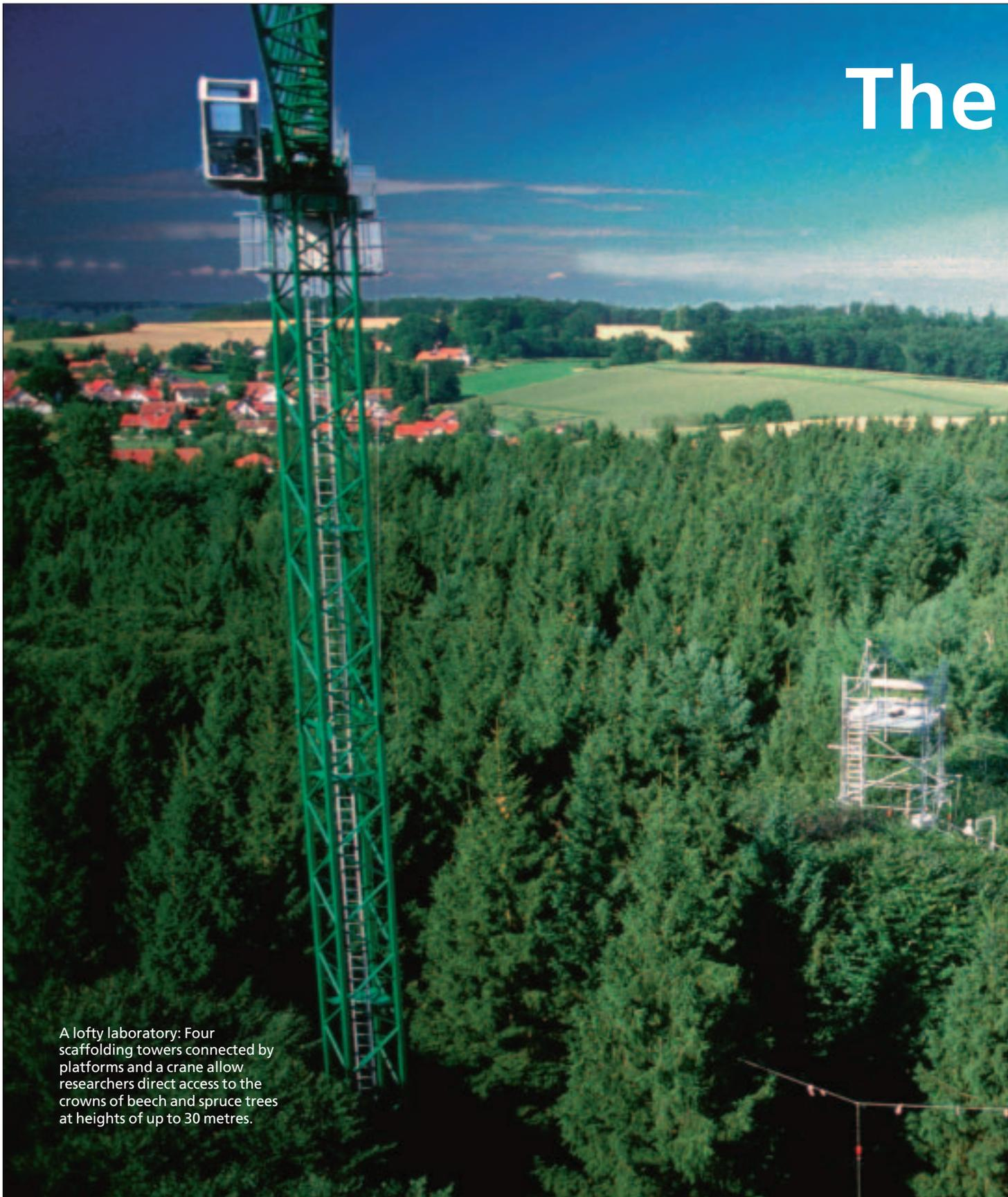
A lofty laboratory: Four scaffolding towers connected by platforms and a crane allow researchers direct access to the crowns of beech and spruce trees at heights of up to 30 metres.
