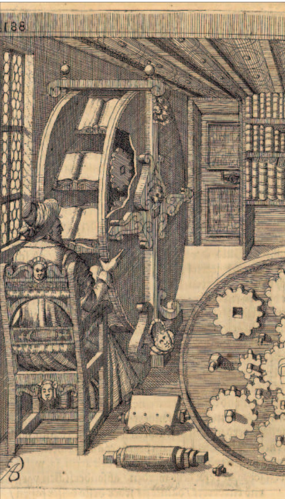
The concept of learning by using hypertext is not a new idea: On this book wheel, designed by Agostino Ramelli in the 16th century, a foot pedal was used to turn a wheel to which books were attached, allowing individual pages and relationships to be found more quickly.
