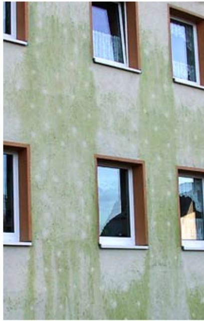
The façade of a block of flats covered in algae. The extra layer of insulation facilitated the unintentional coloration. If sufficient water is available, what starts off as a gradual colonisation by microalgae can rapidly turn into a "green skin", as seen on the stone statue below.
