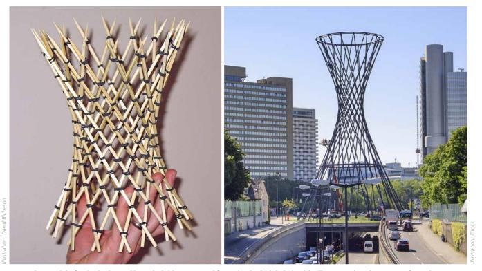
A wooden model of a single-sheeted hyperboloid constructed from simple shish kebab sticks illustrates that there are surfaces that are entirely curved but which still have an infinite number of straight lines on their surface. Right: Mae West sculpture in Munich-Bogenhausen.
